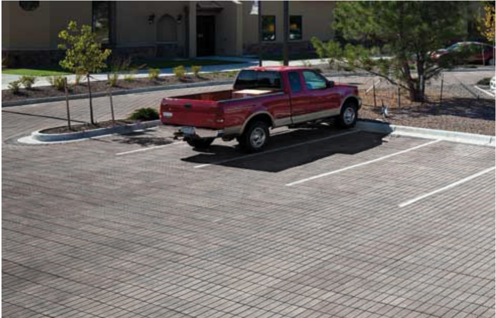
SOUTHERN PLAZA/PARKING AREA PAVEMENT
