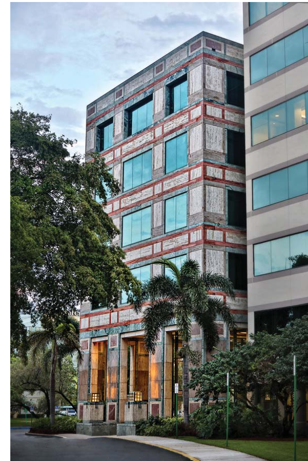
BUILDING ENTRY AT EXISTING OFFICE 3750 NW 87TH AVENUE
