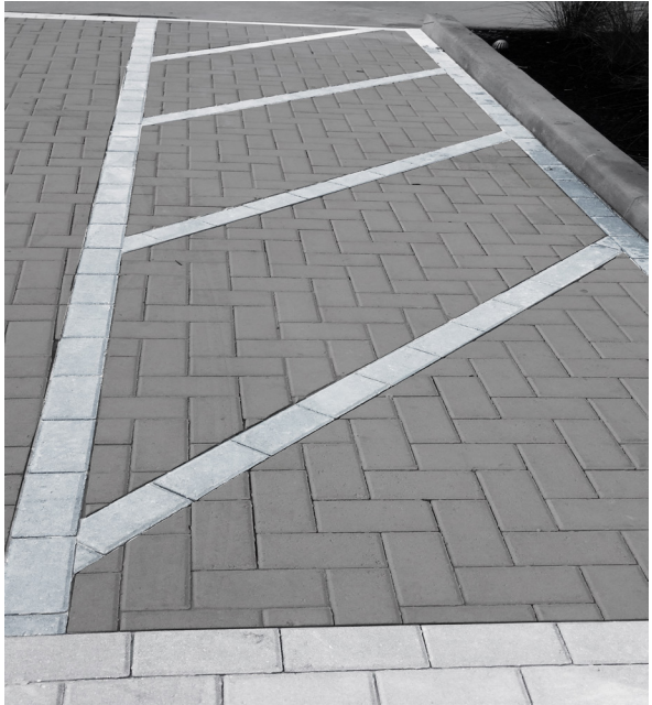
PARKING AREA PAVEMENT
