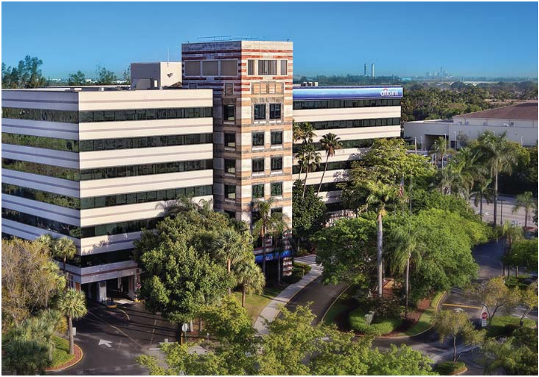
EXISTING OFFICE BUILDING AT DORAL BOULEVARD
