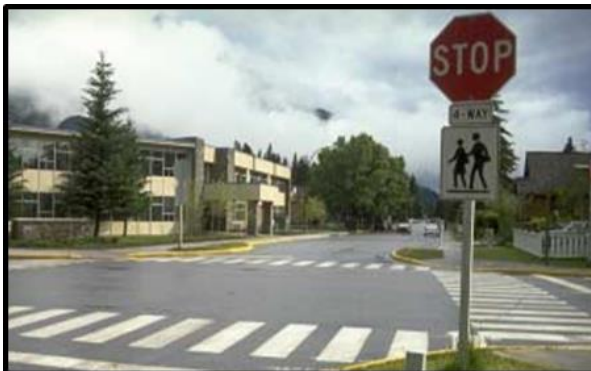
Example of High Visibility Crosswalks
