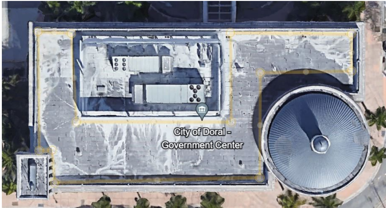
Figure 1. Aerial Image of the Recommended PV System Area
