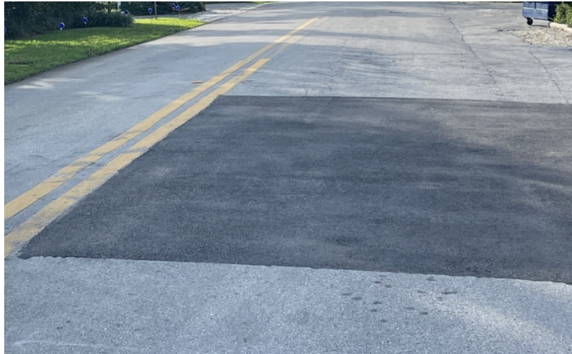
Figure 12. Roadways showing pavement patching
