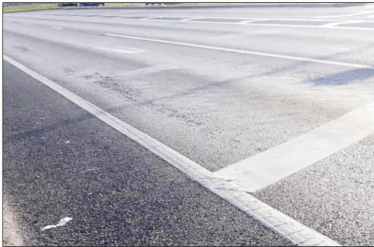
Figure 6. Light rutting
