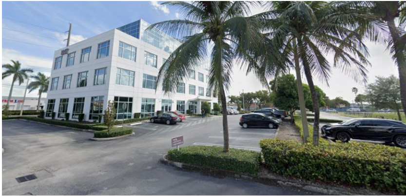
Image 1. Northwest corner of the property
