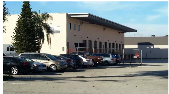
Repetitive Loss Area 11 – Inside of building is elevated
