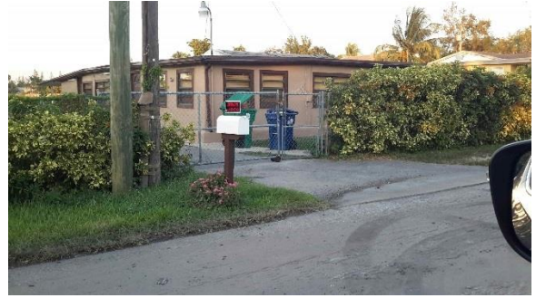
Repetitive Loss Area 21 - House below grade
