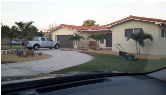
Repetitive Loss Area 20 - Road and driveway slope toward house
