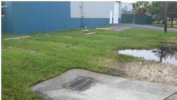
Repetitive Loss Area 1 - Water ponding in lot and not reaching drainage inlet
