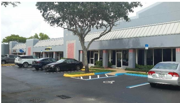
Repetitive Loss Area 15 – Building at grade; parking lot is sloped to catch and drain water
