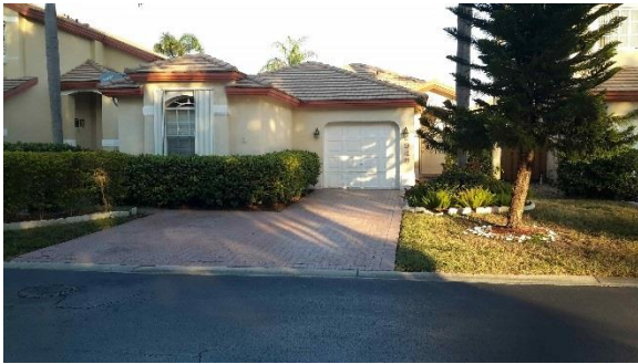
Repetitive Loss Area 19 - House at grade without guttering
