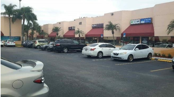
Repetitive Loss Area 7 – Building at grade; water could enter easily from parking lot
