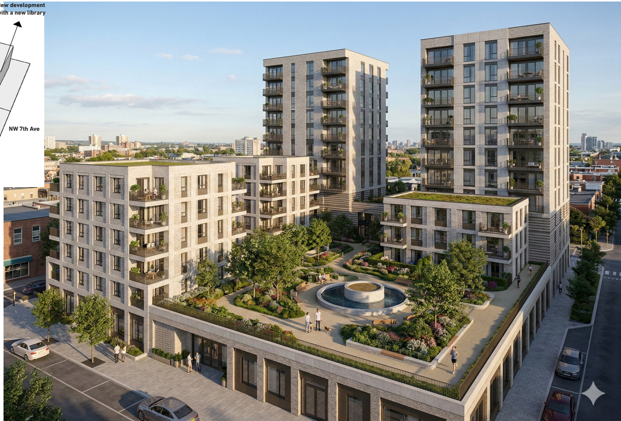
Proposed redevelopment and new overlay district on public property that retains civic uses including library and police station with a residential component..
