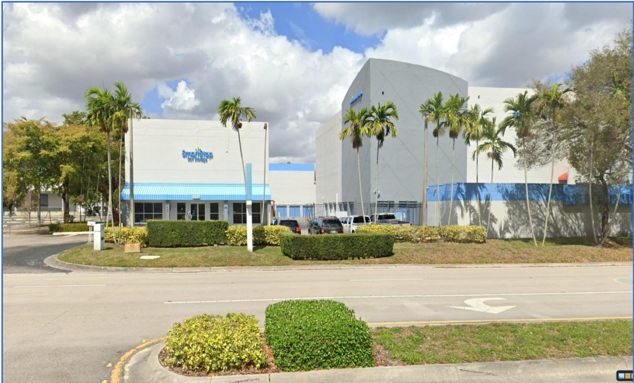
Image I. View from the South
