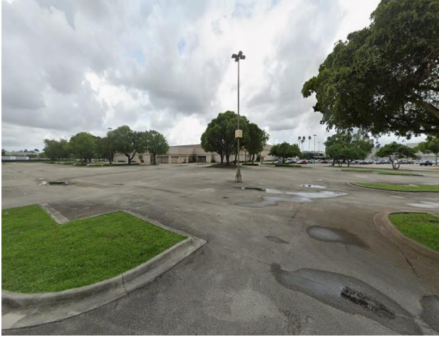
Image 1. Northwest corner of the property
