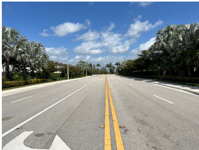
Figure 15 NW 102 nd Avenue looking north towards NW 90 th Street
