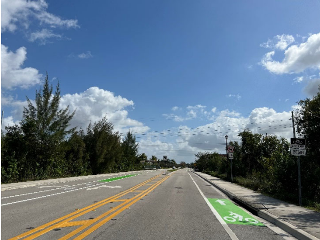
Figure 13 NW 88 th Street looking east towards Central Park
