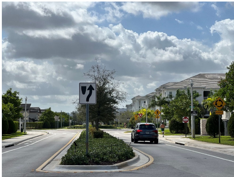
Figure 8 NW 104 th Avenue looking south at the NW 78 th Street roundabout
