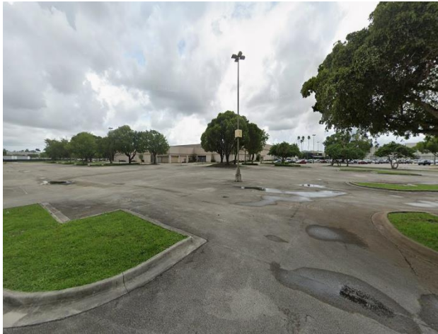
Image 1. Northwest corner of the property
