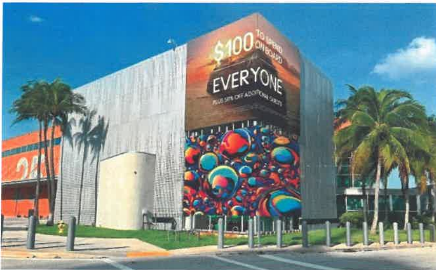
Port Everglades/ Terminal 25 Primary Entrance Feature
