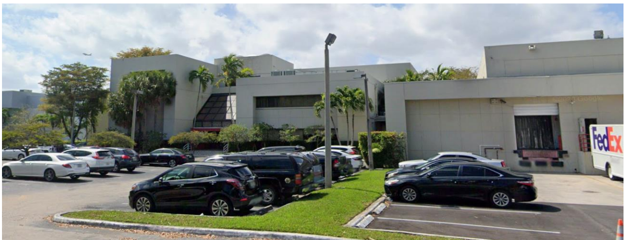
Image 4. View of existing office building to be demolished on south portion of property
