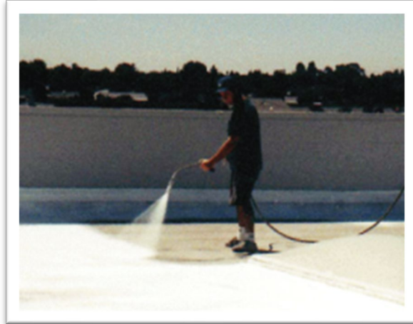
Figure 6. Cool coating being sprayed onto a rooftop
